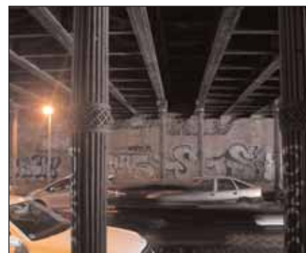
Blick quer zur Fahrbahn
